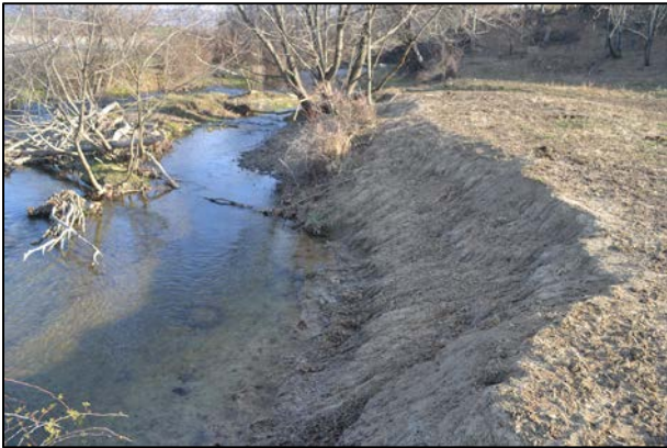
BEFORE: Severe stream degradation from unrestricted livestock access
