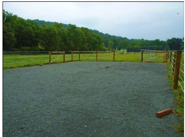
After – Roofed manure stacking pad (not picture liquid manure storage)
