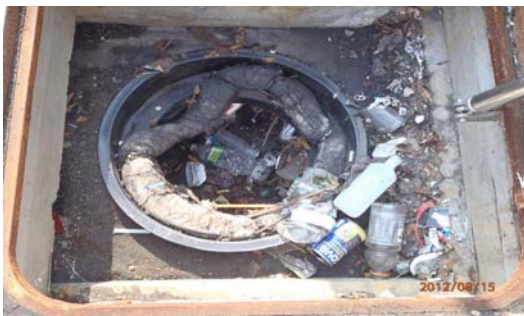
Terre Urban Protector Pretreatment Prevents Constant Urban Eyesore Maintain 2' x 4' Area Extends Useful Life of Rain Garden
