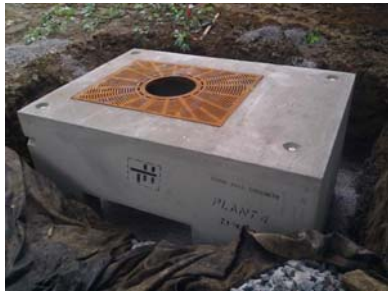
Terre Tree Filter Structure
