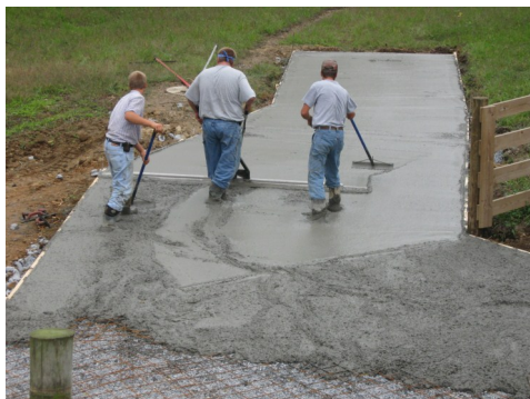
Workers Install an Animal Walkway—One of many Important BMPs
