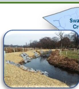
Through a SRRF grant, the BCCD was able to install over 300 ft. of streambank protection on the Irish Creek that was also planted in a CREP Riparian Forested Buffer.
