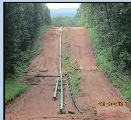
Before: Trenching for the Pipeline; grading after pipe has been installed.
