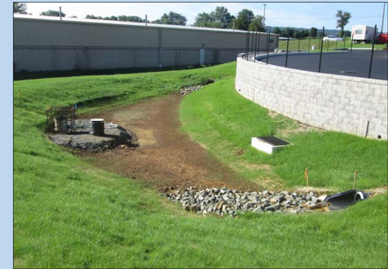
Top Image: Temporary sediment trap
