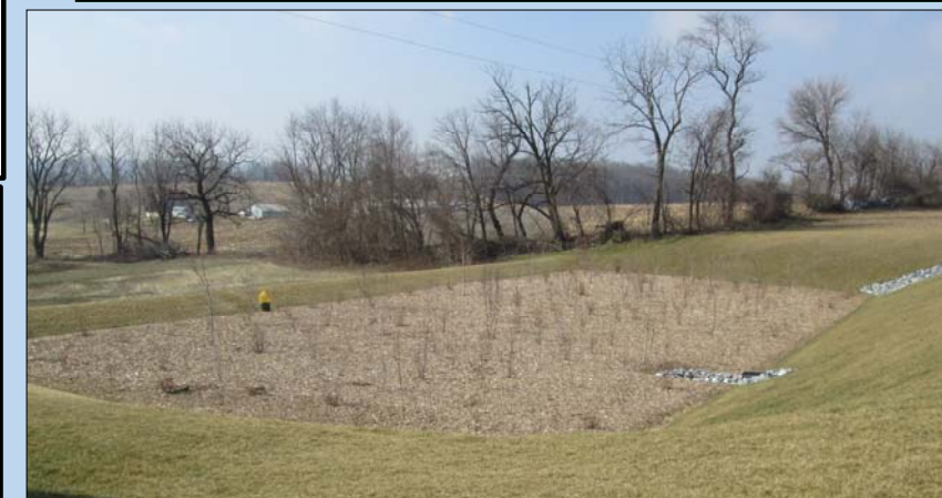
Bottom Image: Completed bio-retention basin
