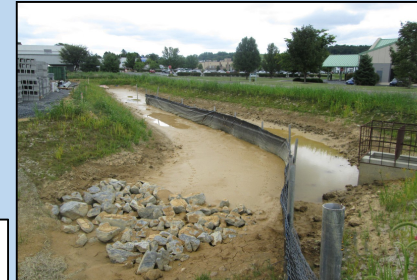
Top Image: Construction of a sediment trap
