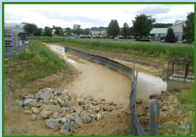
Top Image: Construction of a sediment trap
